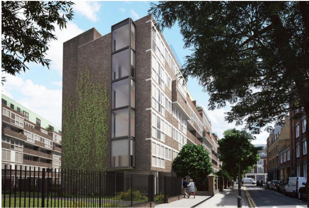
Compton Street Block overlooking Compton Park
